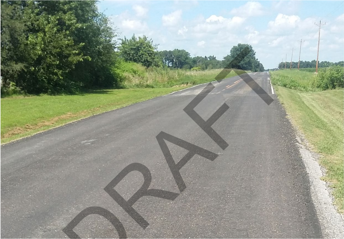
Typical asphalt pavement repair
