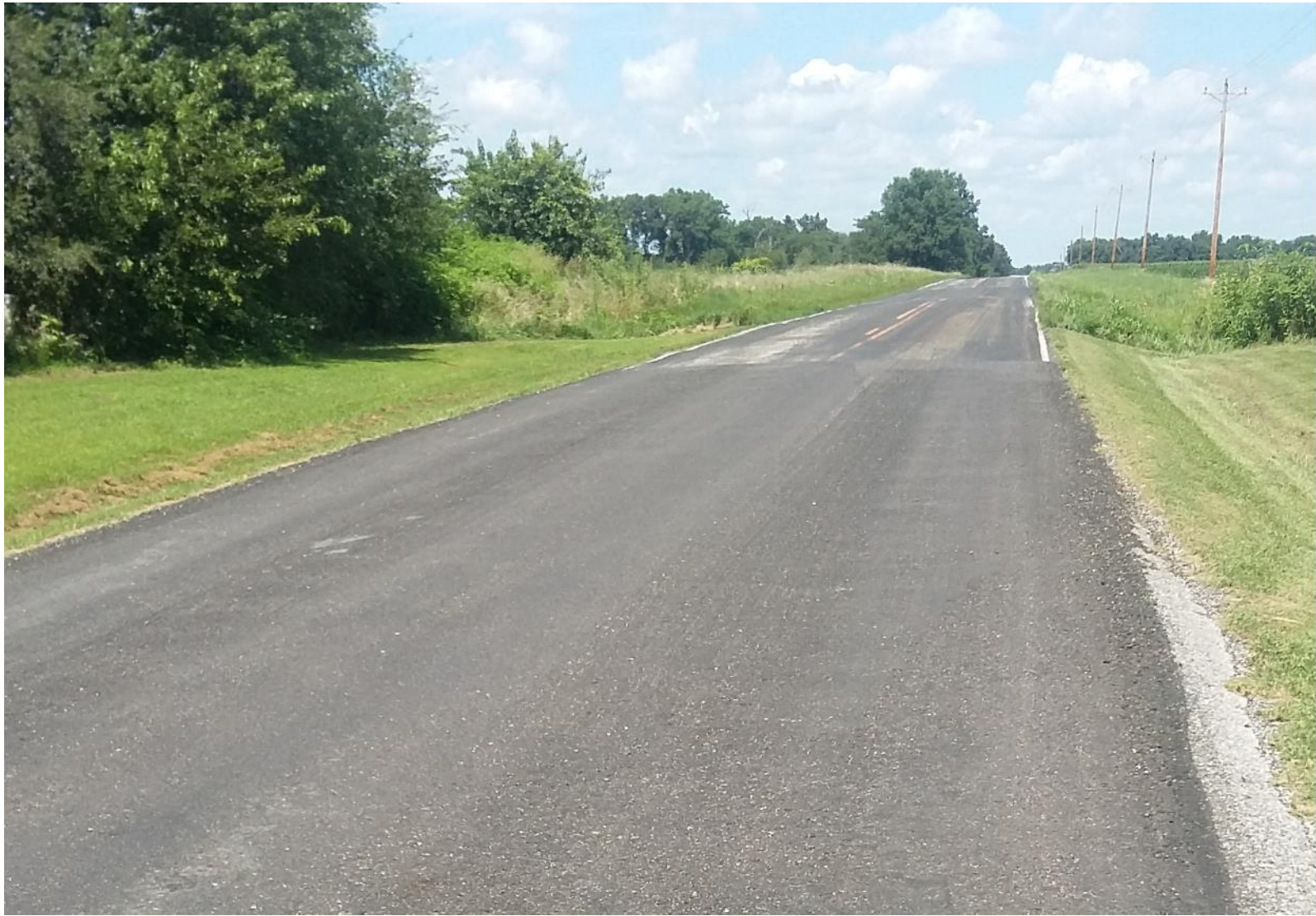
Typical asphalt pavement repair
