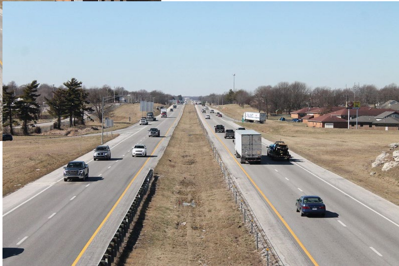
Truck traffic on I-44 through Springfield, MO, showing stretches with no center median barrier, and the grassy median where the additional lanes will be constructed. Even minor accidents can shut down both lanes of the roadway creating significant delays.
