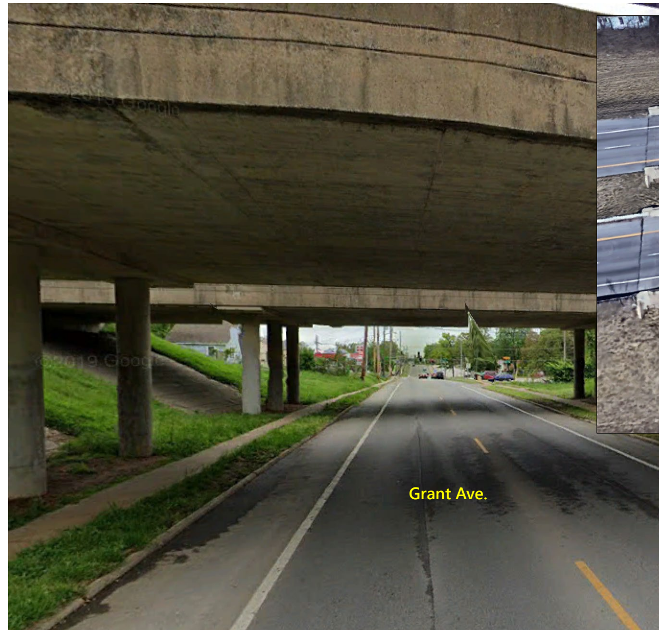
I-44 Bridge (notice the twin bridge design) – two lanes in each direction – over Grant Avenue. Close-up view. Left Photo: Underbelly view. Right Photo: Aerial View of same twin bridge design. The FIX I-44 project proposes to reconstruct three, two-lane twin design bridges on I-44.
