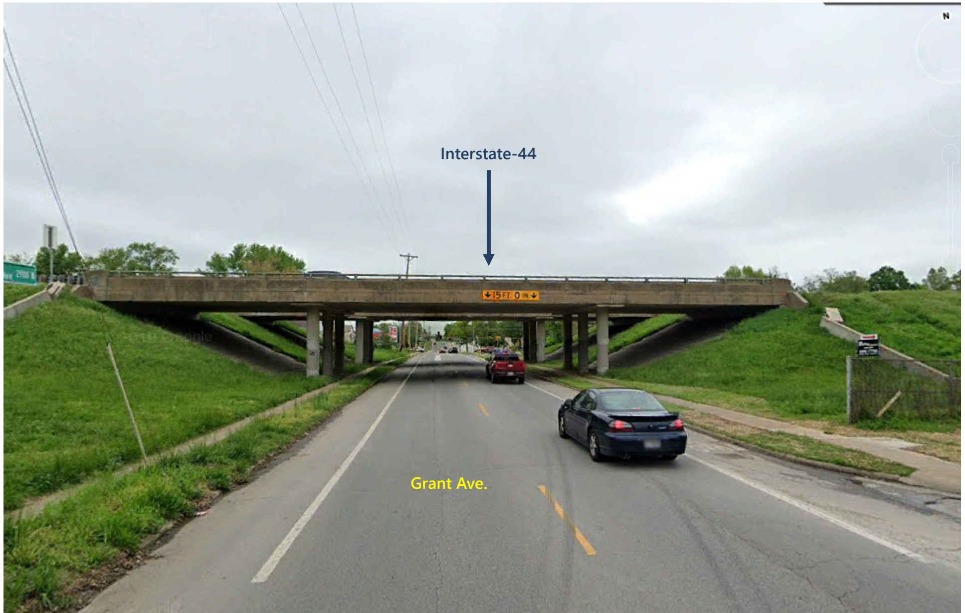
This is one of three two-lane bridges that will be reconstructed. The surface street is Grant Ave.
