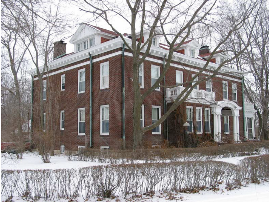
view to NE, brick house
