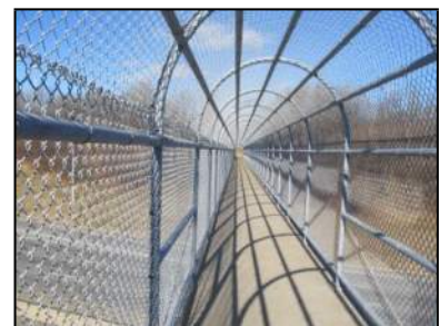
Pedestrian Bridge West of Lister Avenue
