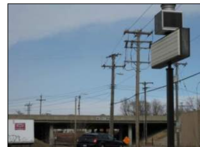
Overhead Power Lines
