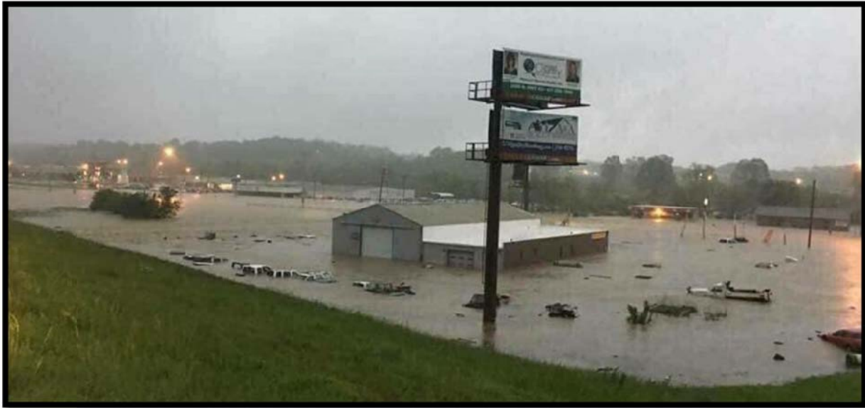
Shown is a view of flooding caused by April 28-29, 2017 storms. Water spilled out from the banks of Howell Creek, which split the city in half and caused millions of dollars of damage. The BNSF rail line and Howell Creek are located at the tree line.
