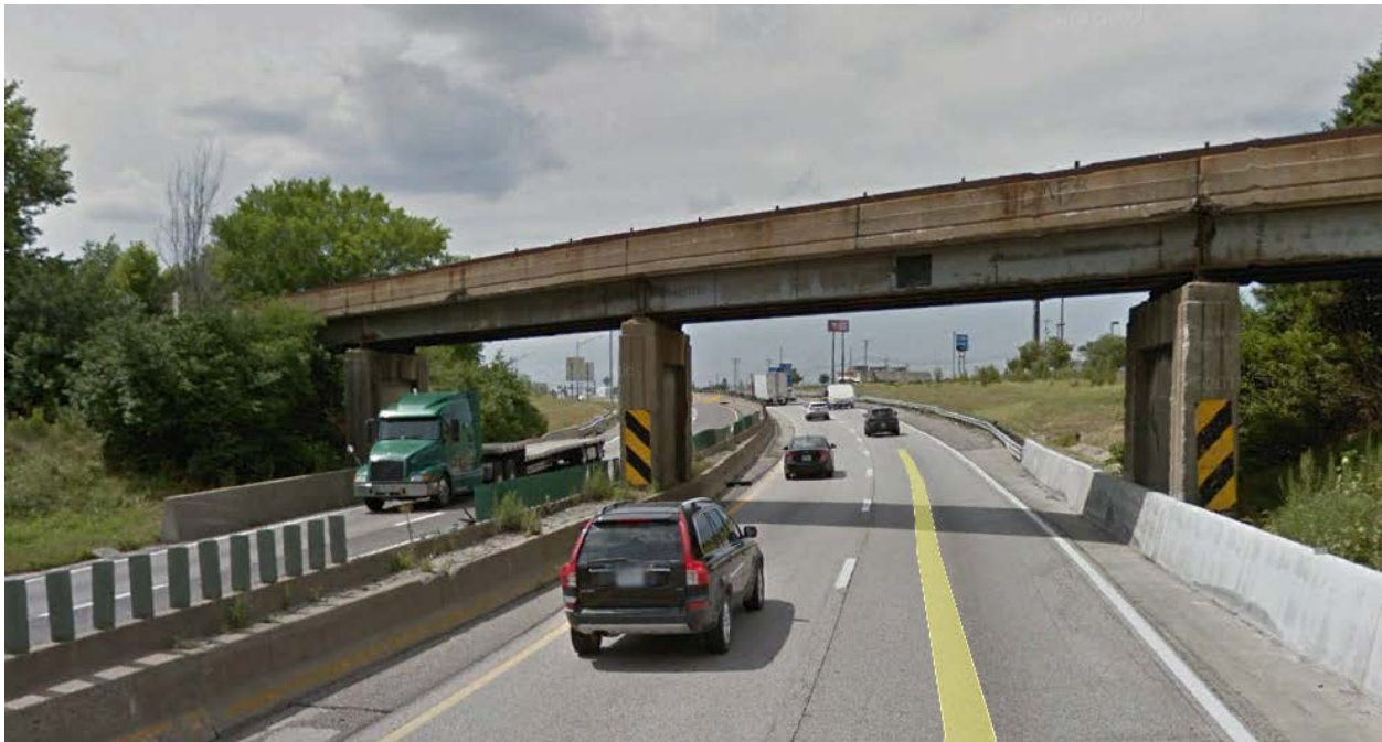
Figure 2 - Existing NSRR Grade Separated Crossing
