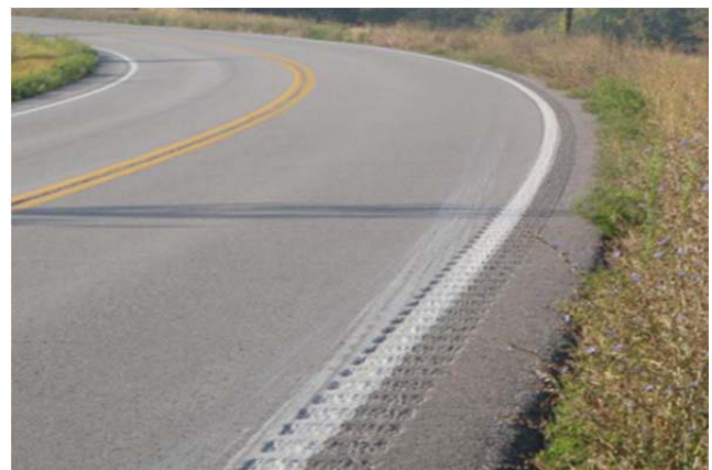
Roadway with Rumble Stripe
