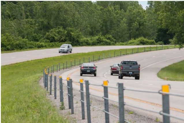
4-Lane Road with Median Guard Cable
