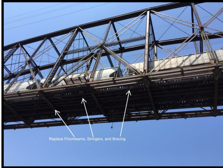
Figure 8: Merchants Bridge Truss Floor System, Floorbeams, Stringers, Bracing
