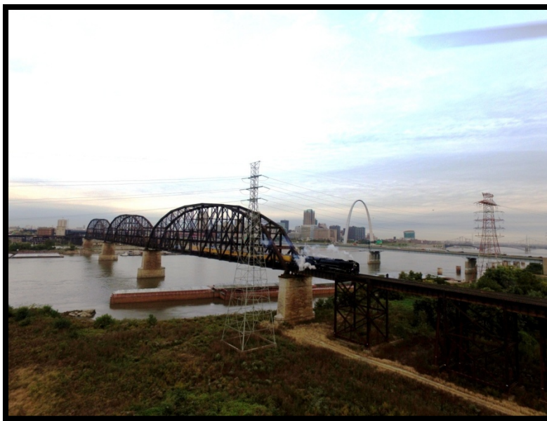
Figure 12 -- MacArthur Bridge looking Northwest
