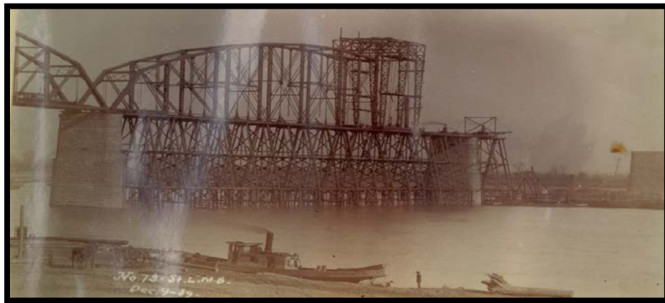
Figure 2-- Merchants Bridge Construction December 9, 1889
