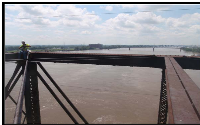
Figure 9 -- Hands-On SGR Inspections
