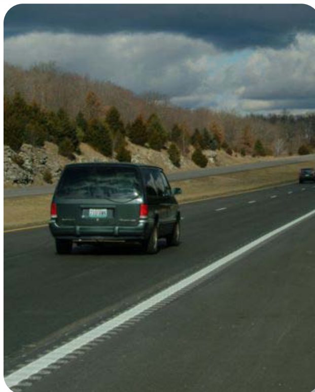
Edgeline Rumble Strips
