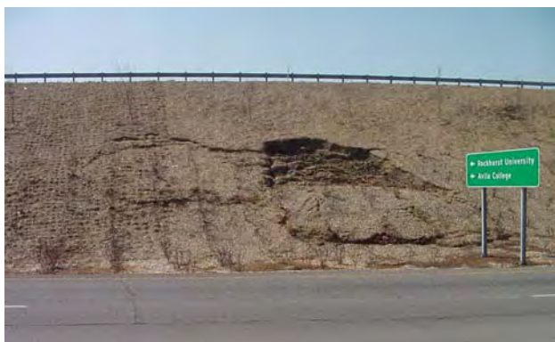
Typical shallow or "nuisance" slide along Missouri roadway.
