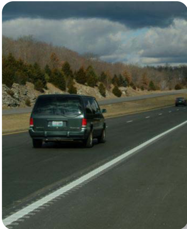
Edgeline Rumble Strips
