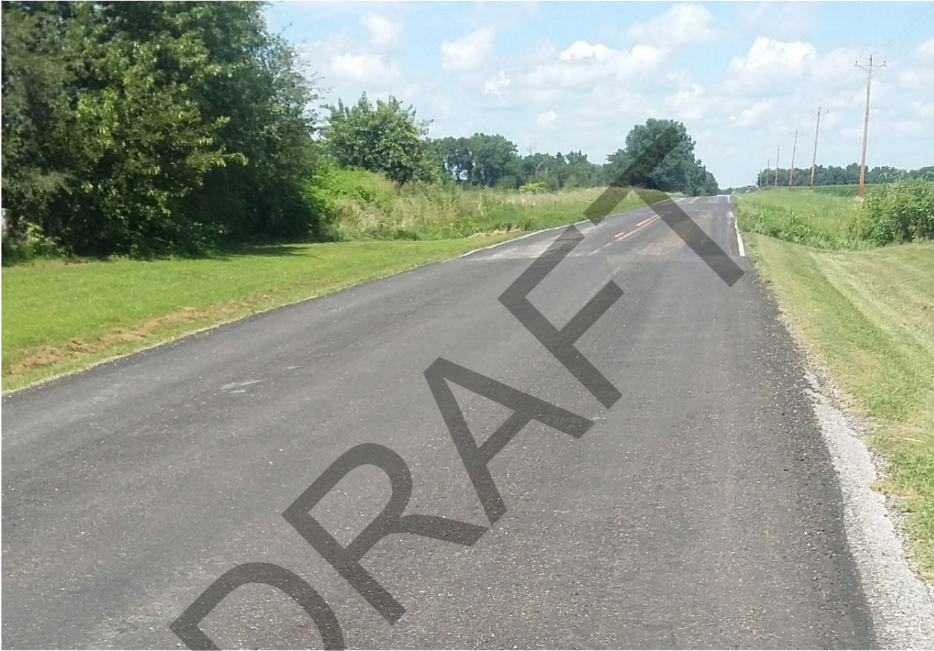
Typical asphalt pavement repair
